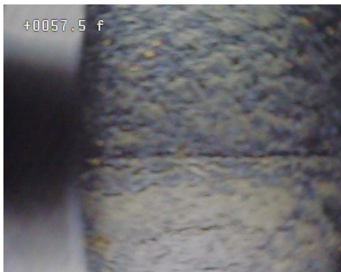
Figure 6: Image of the casing joint under water at 55.8 ft-bls (57.5 feet from top of casing). As discussed previously in the Well Details section, the depth of this joint is what suggests there is most likely more casing below the current bottom of the well at 65.41 ft-bls.
