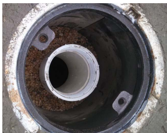
Figure 34: Photo of 6-inch steel casing reduced to 4-inch PVC and raised closer to land surface.
