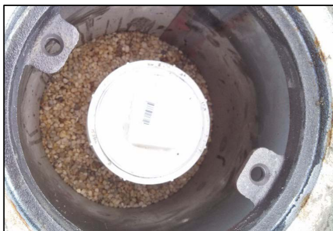
Figure 35: Annular space filled with pea-gravel and new protective flush-mount cover cemented in place.
