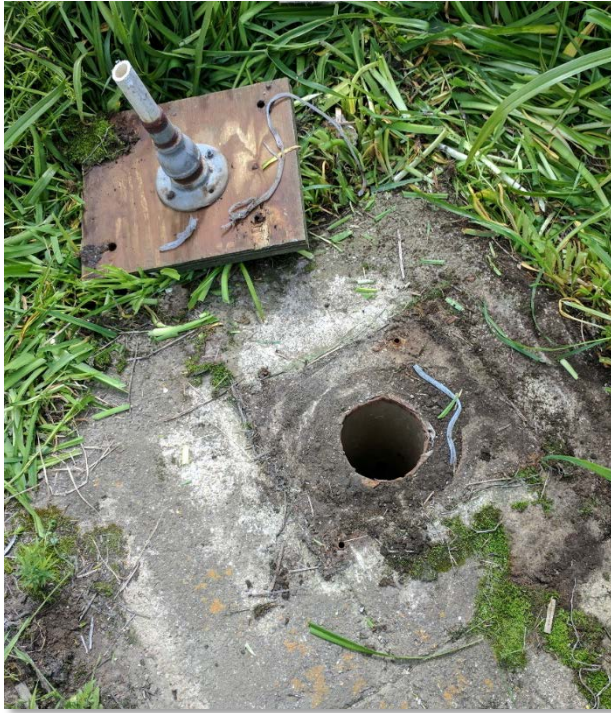
Figure 13: Photo of current well access displaying need for installation of a protective cover.
