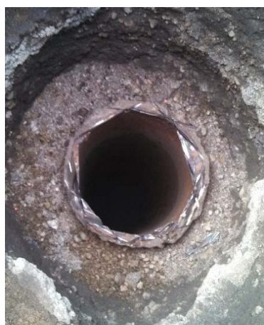
Figure 33: Well after the angle grinding was completed.
