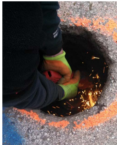
Figure 32: Angle grinder being used to cut through steel plate on well.
