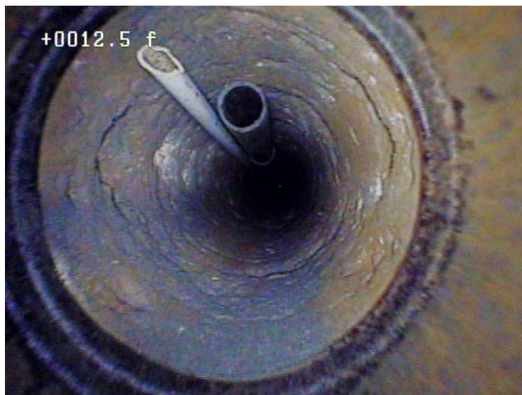
Figure 9: Video log image of the bottom of the casing with the two pipes sitting inside the well. The casing stops at 13.2 ft-bls and the pipes start at 13.4 ft-bls.
