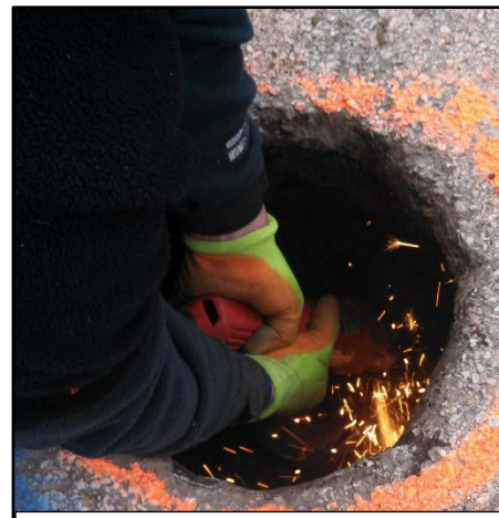
Angle grinder used to cut through steel plate on well
