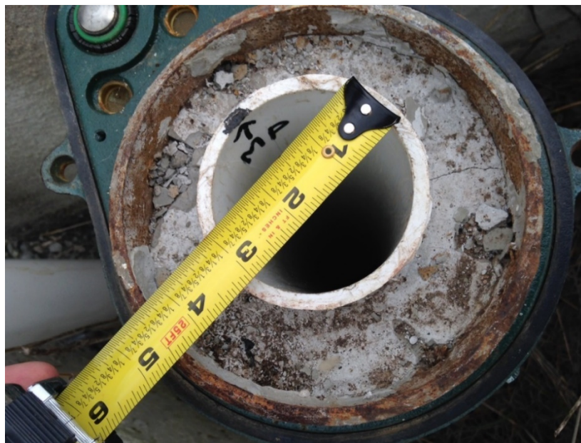
Figure 43: Photo showing the 3-inch pipe (called liner elsewhere) installed within the original casing.
