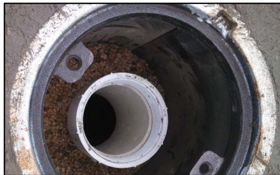
6" steel casing reduced to 4" PVC and raised closer to land-surface
