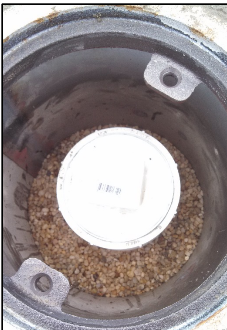
Annular space filled with pea-gravel and new protective flush-mount cemented in place
