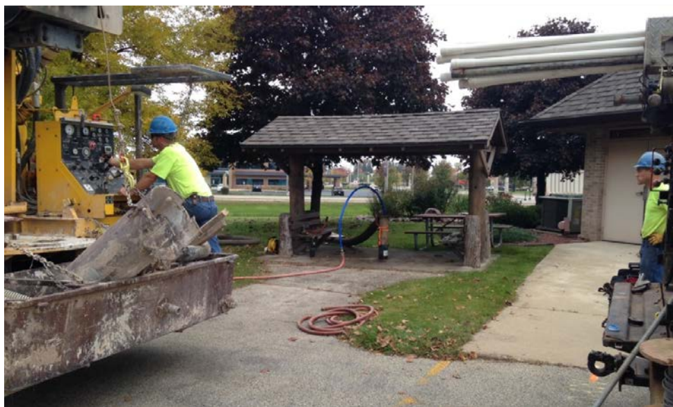
Figure 21: Photo of the air lift process.
