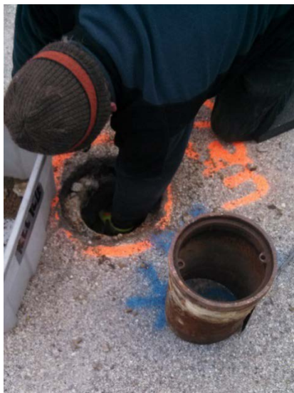
Figure 30: Removal of existing protective flush-mount.
