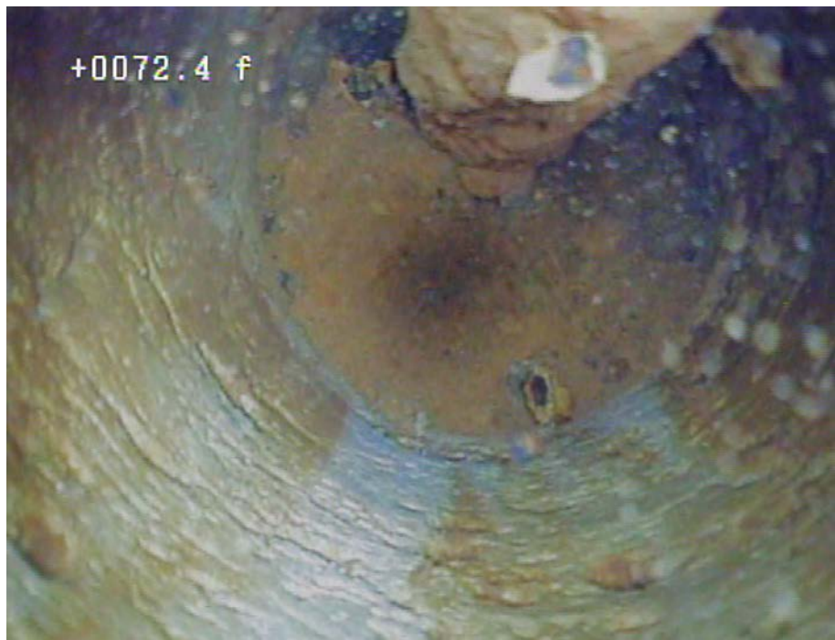
Figure 11: Video log image at the bottom of the well. The PVC pipe is behind the metal pipe in this image.
