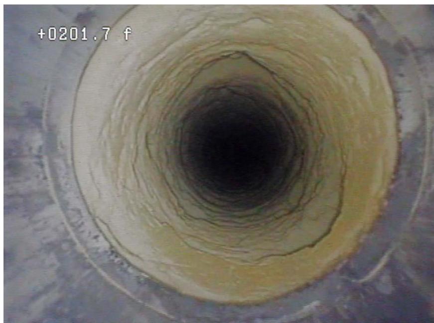
Figure 50: Base of steel casing showing good contact with the carbonate bedrock. Casing and borehole wall appear clean.
