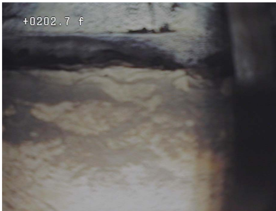
Figure 51: Base of steel casing side view at 202 ft-bls.
