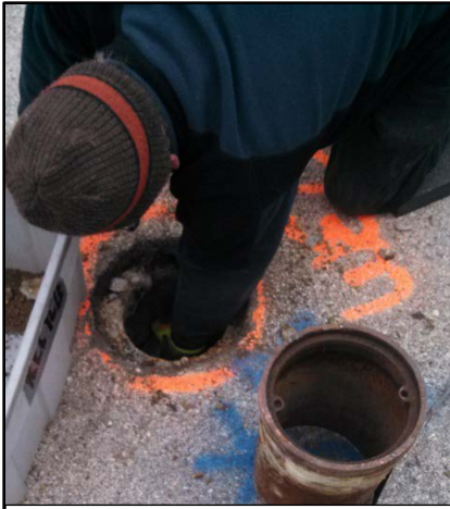
Removed existing protective flush-mount
